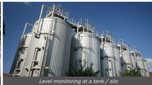
Level monitoring at a tank / silo
