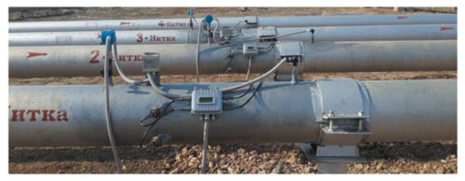
Hot-tapping device for installation of sensors in pipelines under pressure Energoflow HSID-01
