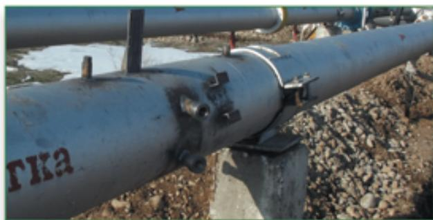
Under order, versions for pressures as high as 250 bar are available. They can also provide for bidirectional flow measurement and thus are suitable for process automation applications.
