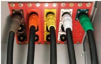
1200 A Cam-Lok power panel with 25% ground ampacity
